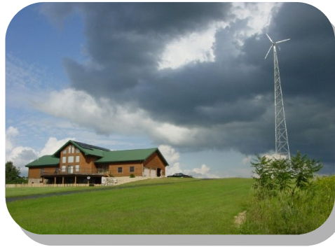
Photo: Small Wind Energy System, Town of Salem, Pierce Co., WI. Roy & Nancy Christianson.
