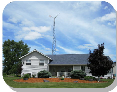
Photo: Small Wind Energy System, Town of Oak Grove, Pierce Co., WI. Bob & Shelley Fleming.
